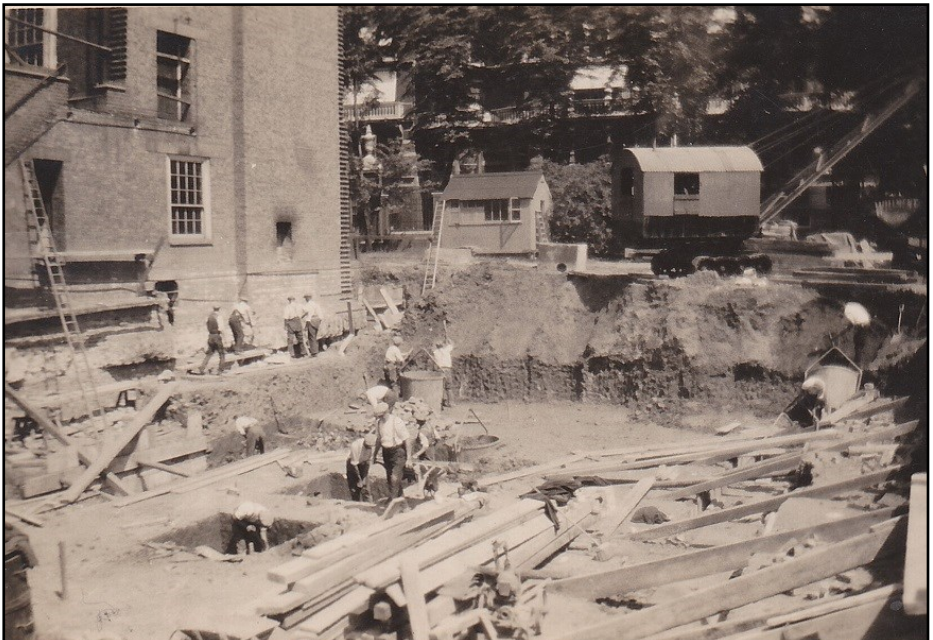
Constructing the Warden's quarters and East Hall, 1930
