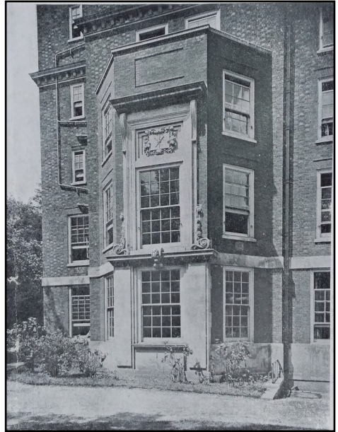
Bay of Hostel Building
